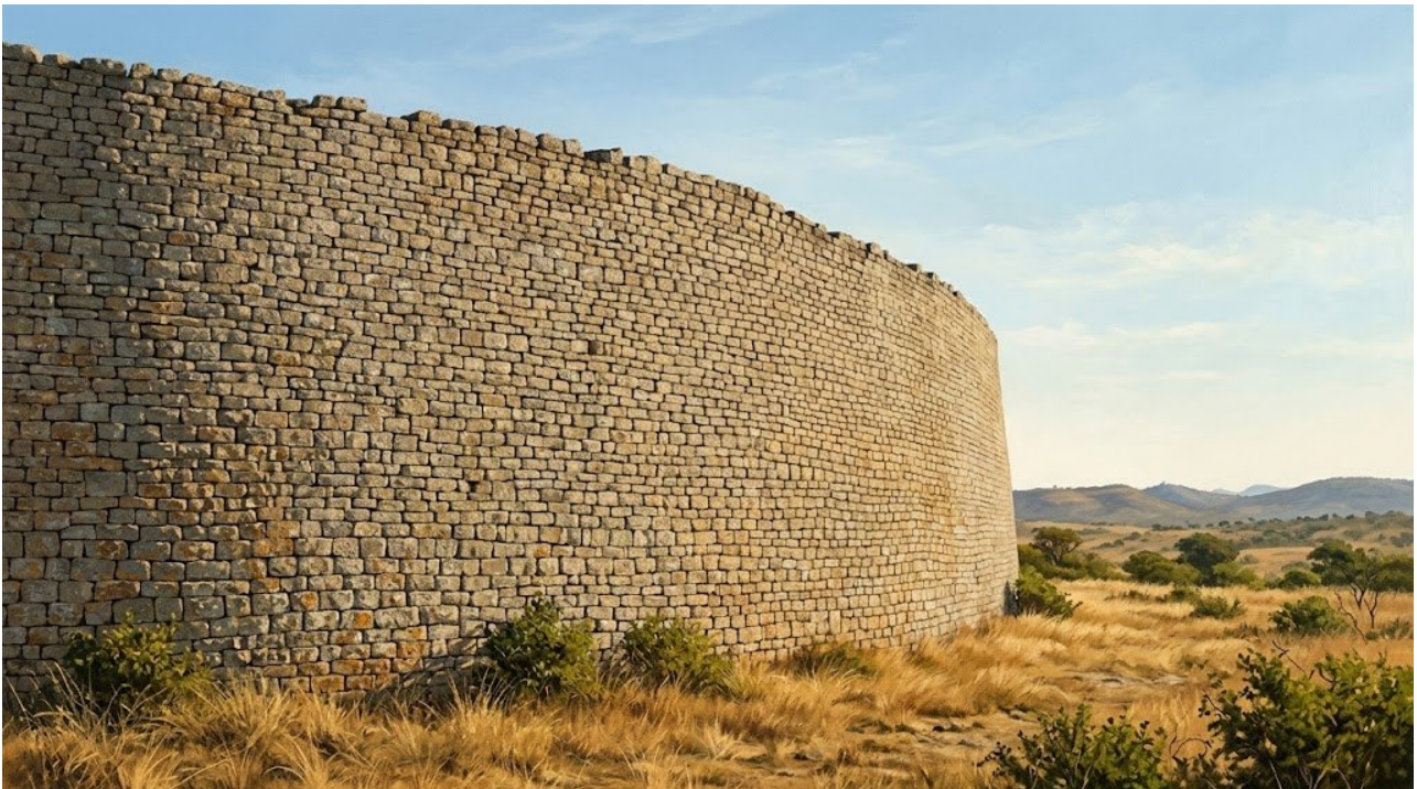
The curved outer wall of the Great Enclosure at Great Zimbabwe, dry stone, no mortar
