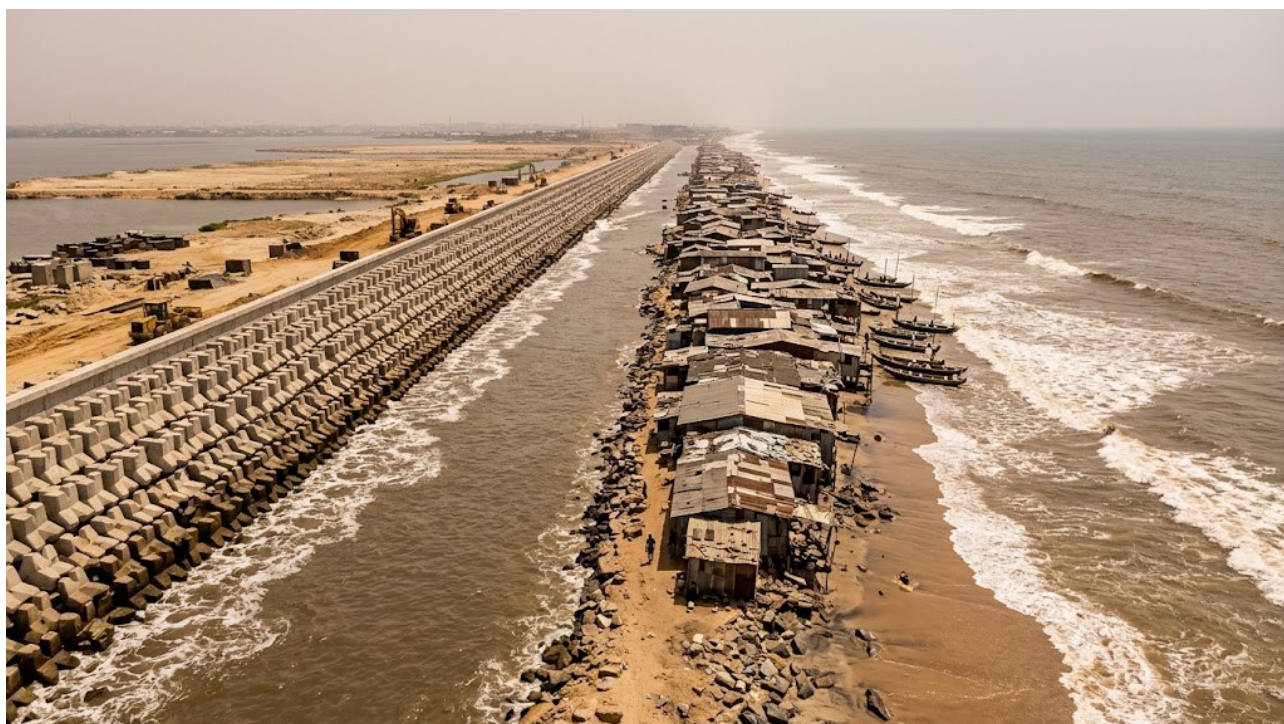
The Atlantic shoreline at Lagos — a concrete revetment on one side, low-lying settlement on the other
